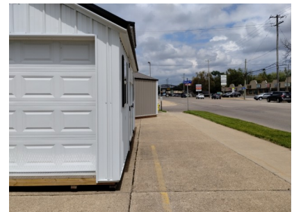
from the left side, looking at where the deck will be located
