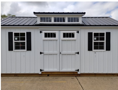
looking straight at where the deck will be located
